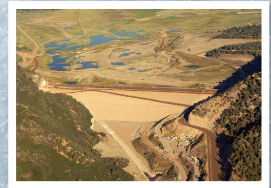
Photo - Ridges Basin Dam Courtesy of Robert Wolff
